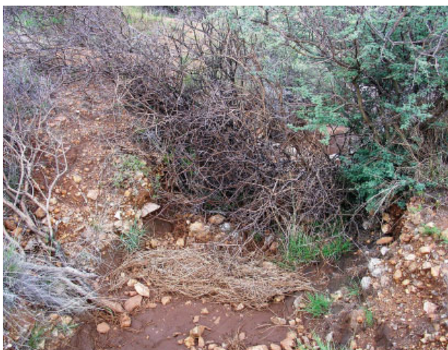
Photo 3: Soil and mulch are trapped on the upslope side of a filter. Photo: Ibo Zimmermann.
