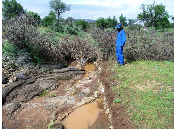
One branch got turned 180° by the water flow, but the wire held it within the filter
