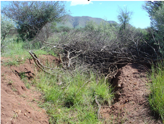
Grasses filter a gully as branches rot
