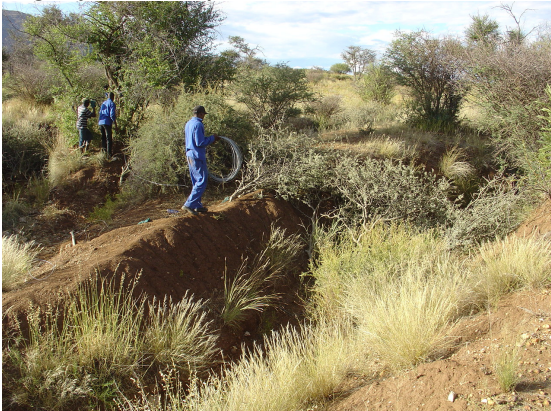
Wire is woven through branches in the filter and tied to nearby trees
